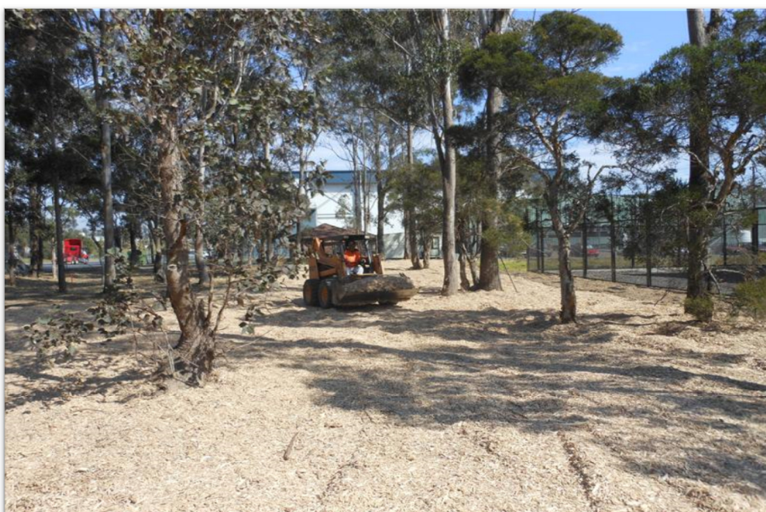
Spreading mulch with a bobcat at the Hoxton Park substation site
